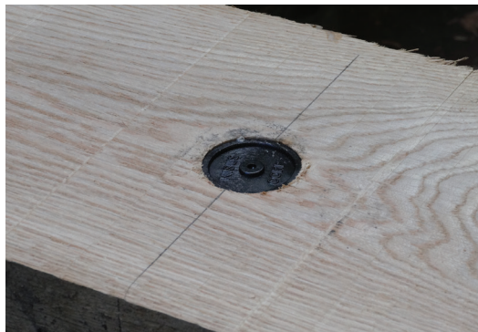
...drilling holes for filling with borate reservoir then plugging.
